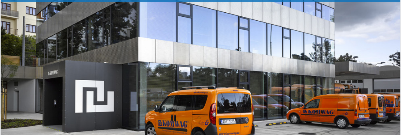
The KOMWAG office building, which opened in 2015, was awarded with a Czech architecture prize.
