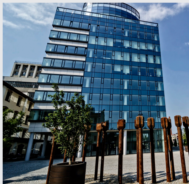
Radisson Collection Belgrade & New Mill Office Building
