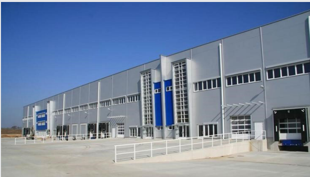
Logistics center Hagenbrunn
